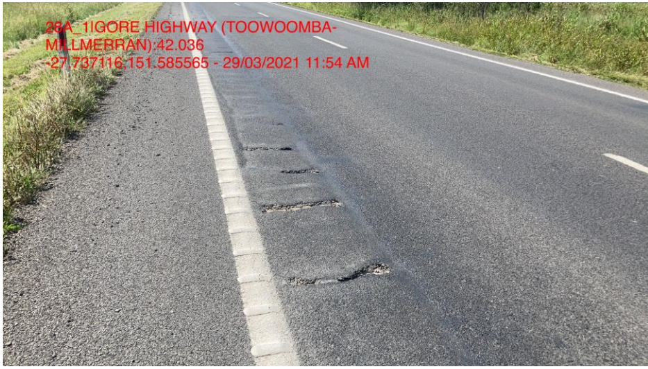
Control section: Double Double only (Right)
