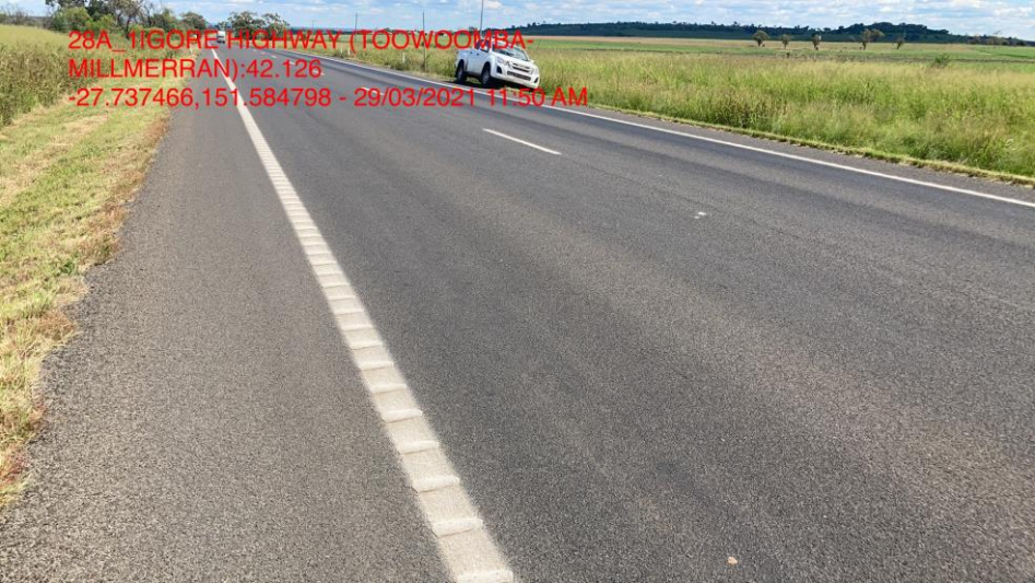
Huesker Chipseal Grid reinforced section (Left)
