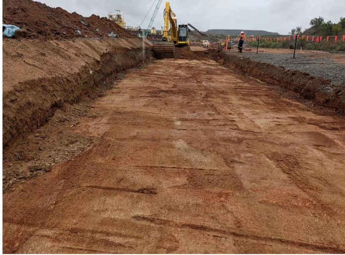
Subgrade Preparation – excavation for ground improvement treatment
