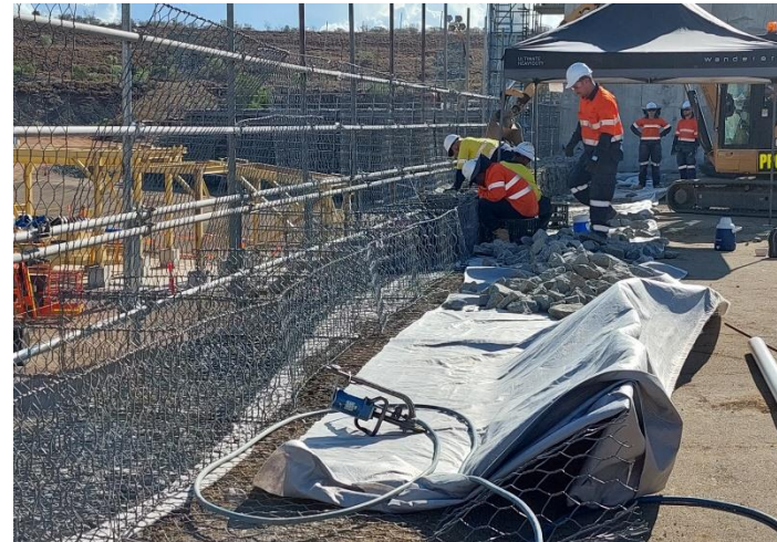
Basket fill stacking prior to framing use
