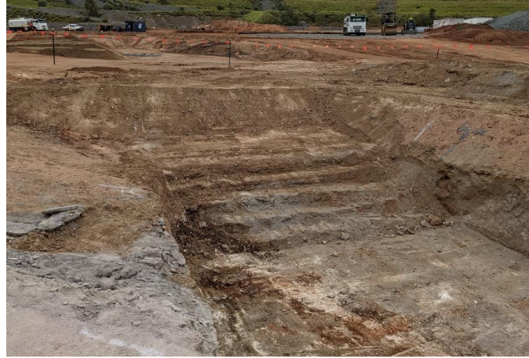
Subgrade Preparation – excavation for ground improvement treatment
