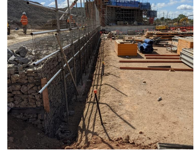
First 1m of ROM wall following Ground Improvement and blinding
