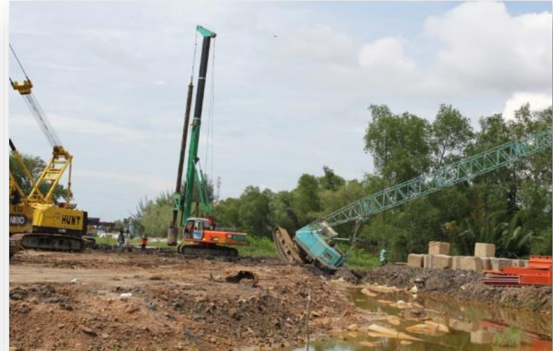
Rotational failure at the edge of platform, Brunei, Asia
