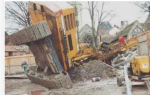
Tilting of the piling rig
