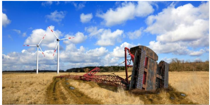
Rotation al failure at the edge of platform
