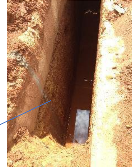
2m deep concrete guide wall
