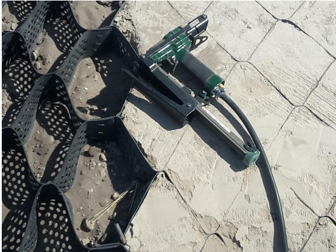
Staple gun for joining of panels
