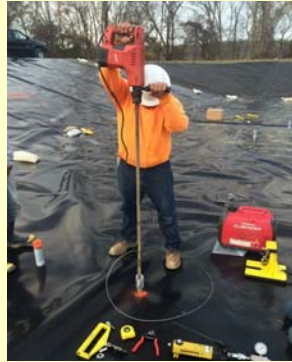
Driving the anchor into soil
