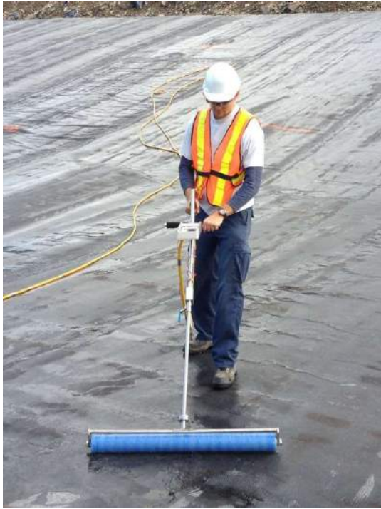
Water Lance Method (ASTM D7002)
