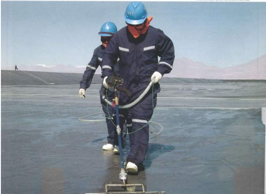
Photo 1 | In constructing the evaporation ponds, after the PVC liner is deployed, electrical leak-detection tests are done (see page 32).
